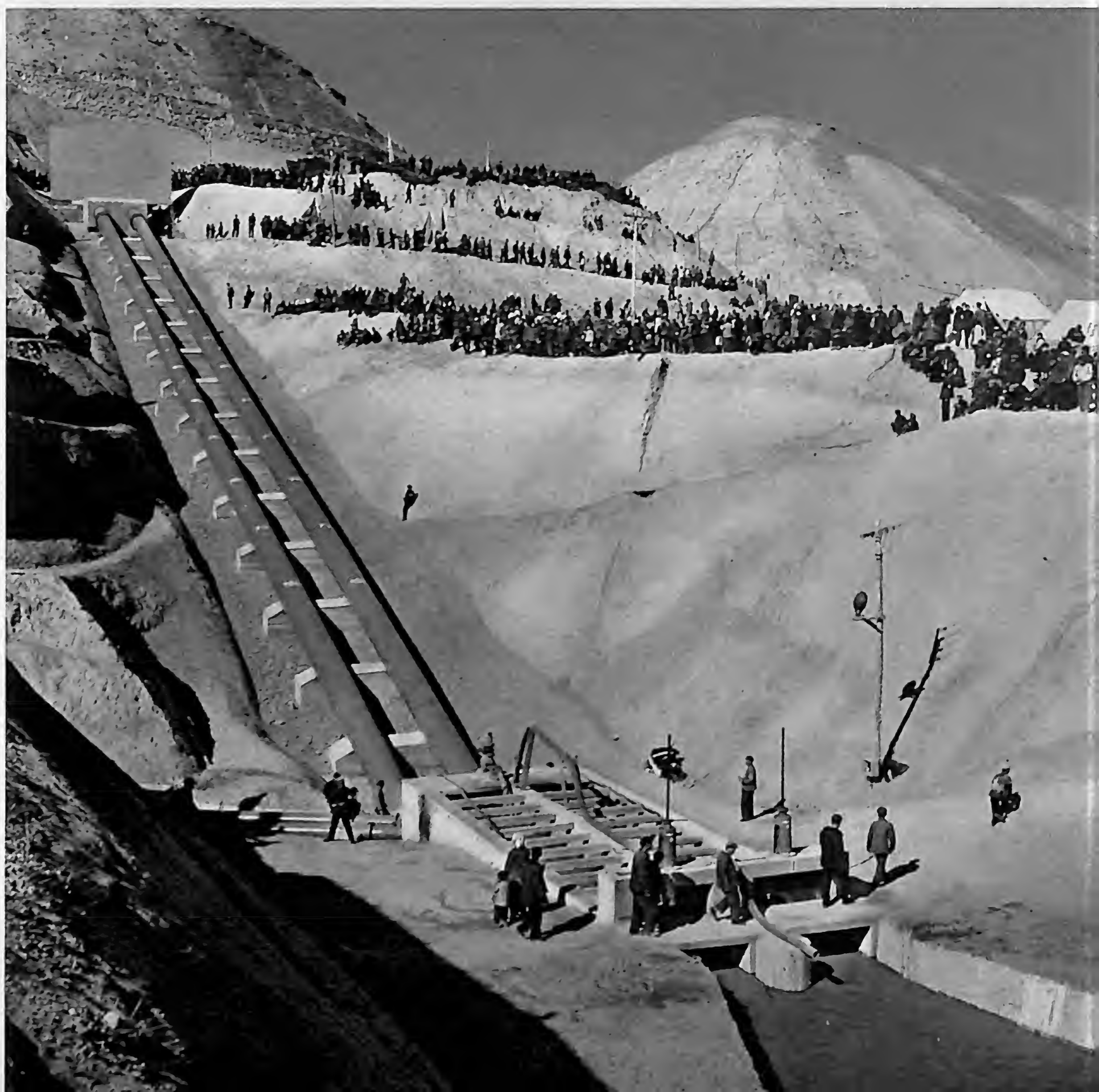
A hydraulic pumping station built by Tatung County. A number of irrigation projects have been completed along the Yellow River and its tributary, the Huangshui River.
